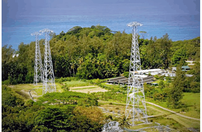
The four steel towers of the former BBC World Service relay station, one as high as 75 metres and the others 65 metres tall, constitute an imposing and familiar feature of Grand Anse. (John Lablache, Seychelles News Agency)
