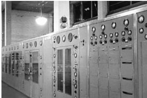
Photo: Rather impressive! The r.f. stages of a 1939 Marconi SWB18 transmitter.
