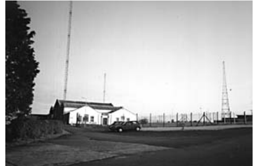
Photo: The original 1925 transmitter building (callsign 5XX) on the left, with the later transmitter building on the far right.
